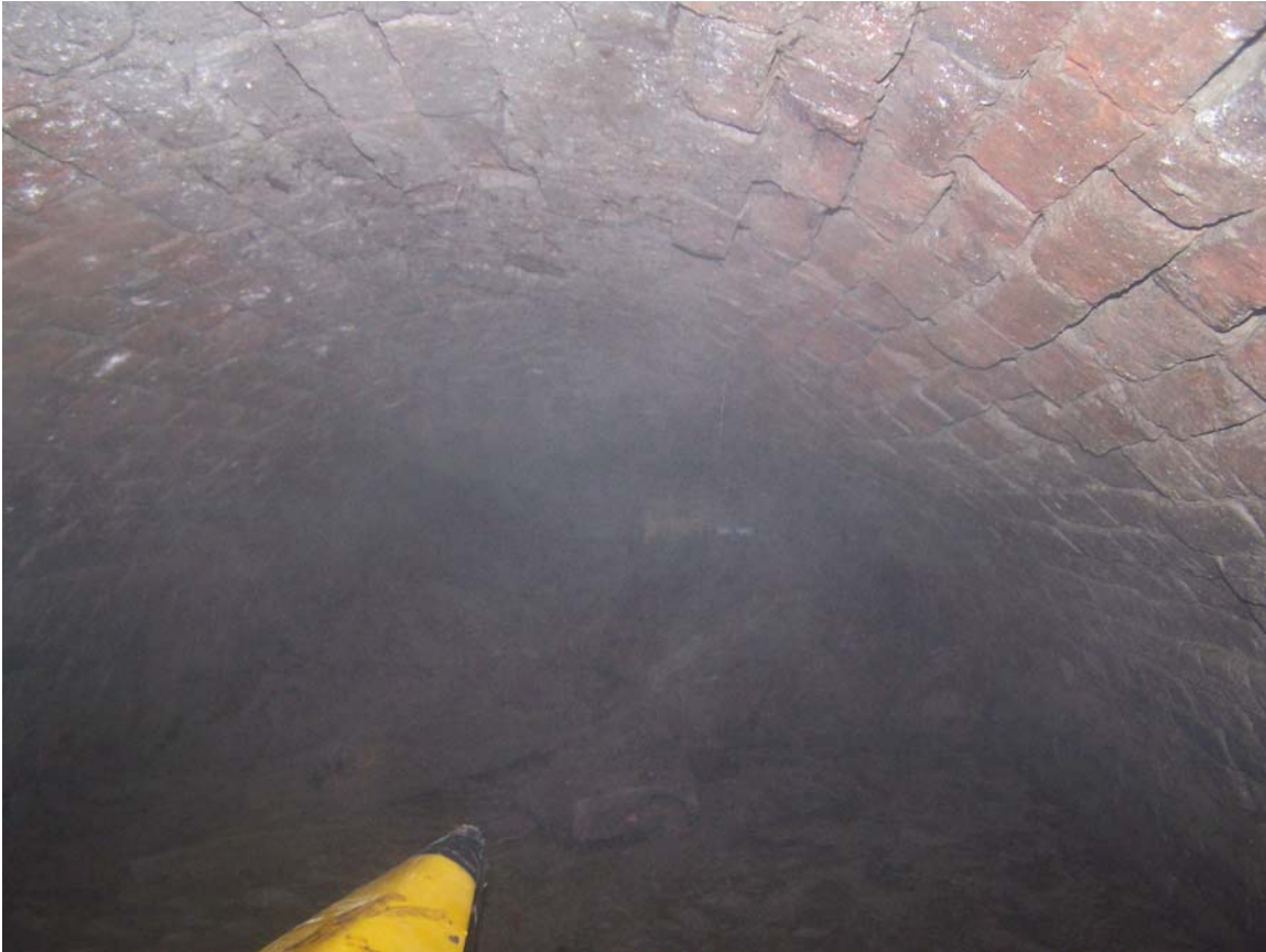
Floor filled with rubble, and the roof quite low.
