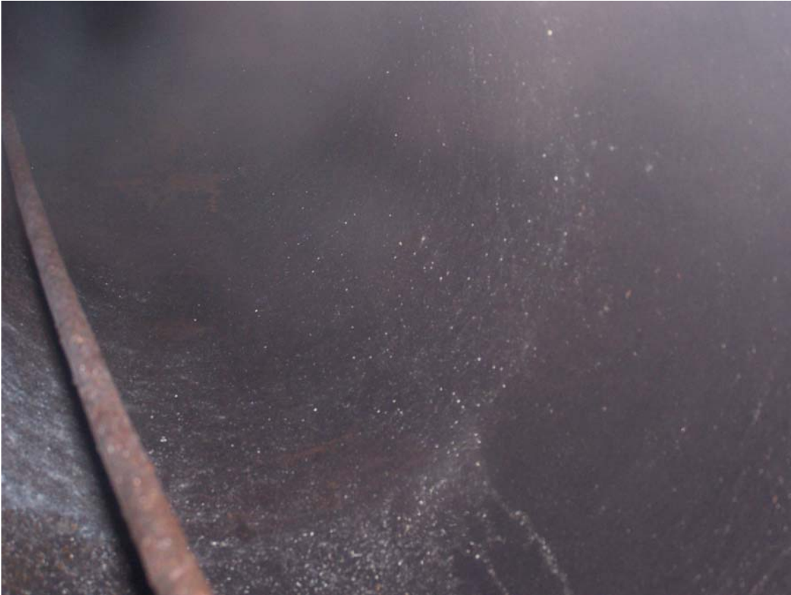
Looking up the entrance shaft of the adit.
