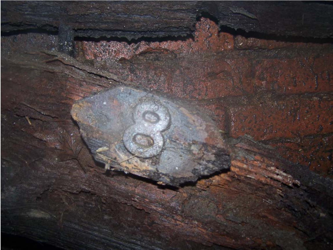
Chain 8 marker is within the third set of shoring. An iron number on a wooden back.
