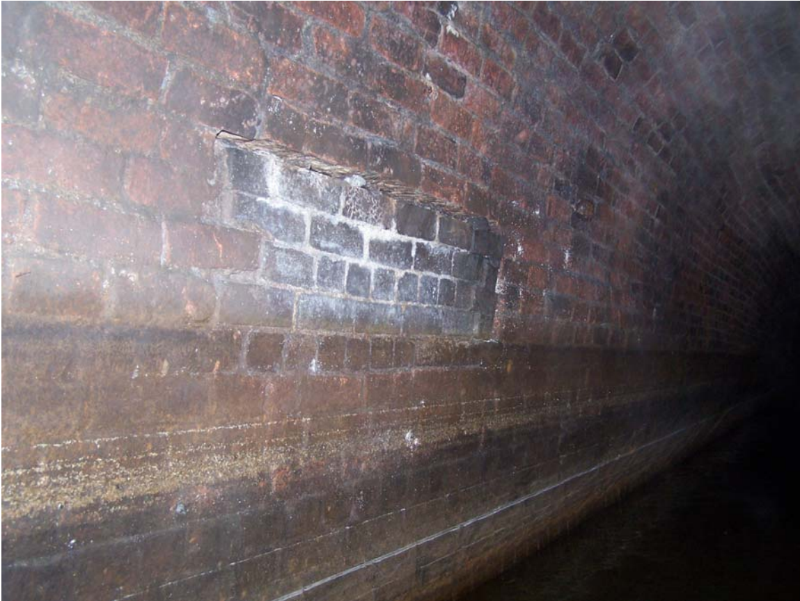
The blue bricks in the centre are a not very well bonded brickwork patch at marker 28. At marker 29 there is water dripping through the roof.
