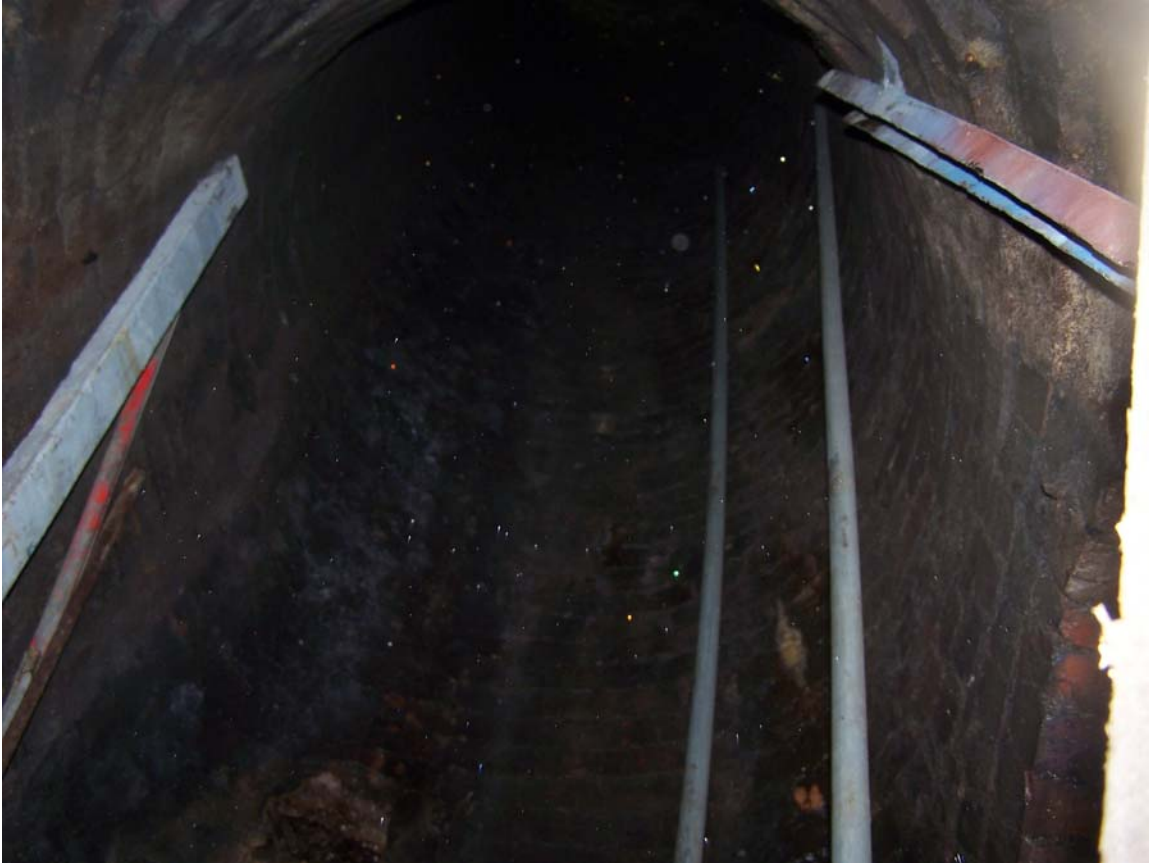
Looking up the airshaft, the items visible are RSJs and scaffold poles which have been thrown into the tunnel.
