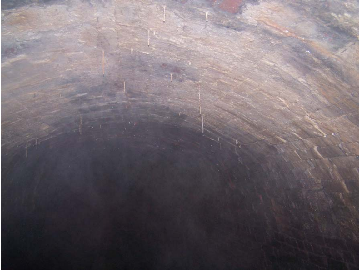
A section without shoring and with straw stalactites at about Chain 4 from the East. The vertical walls near to water/silt level are bowed inwards.
