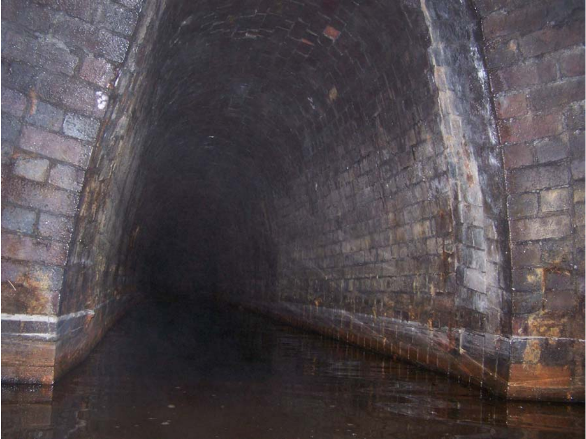
The adit from the tunnel
