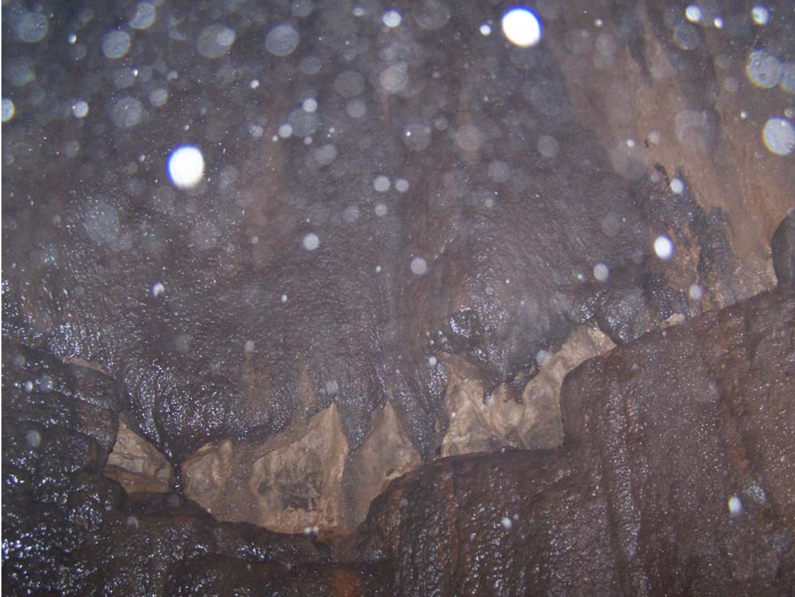
This is a view of the wall of the blast receiver shaft labelled 'I' in the diagram.
