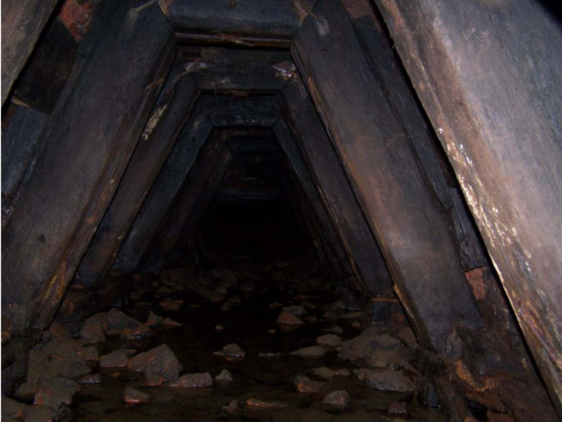
Shortly after the Wide Hole the floor of the tunnel is built up with rubble and the roof is heavily shored up.
