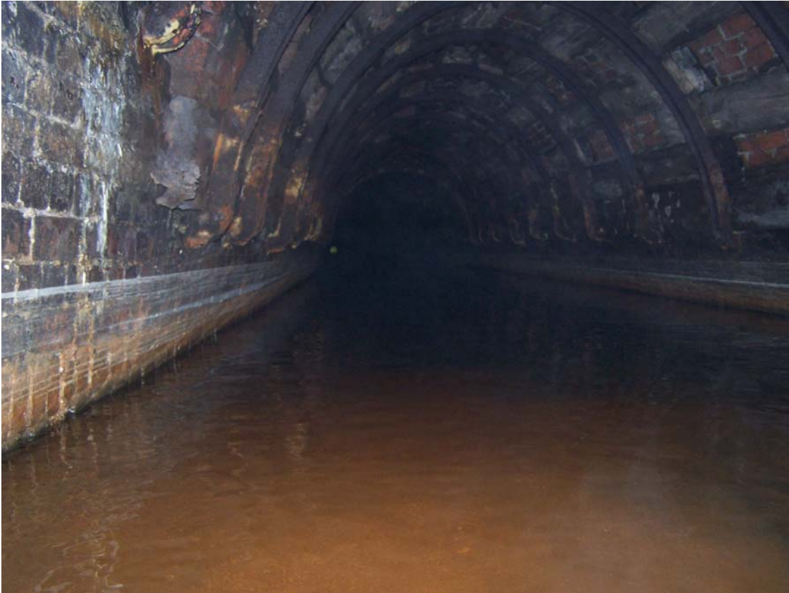
Looking back towards the light of the Western Portal.
