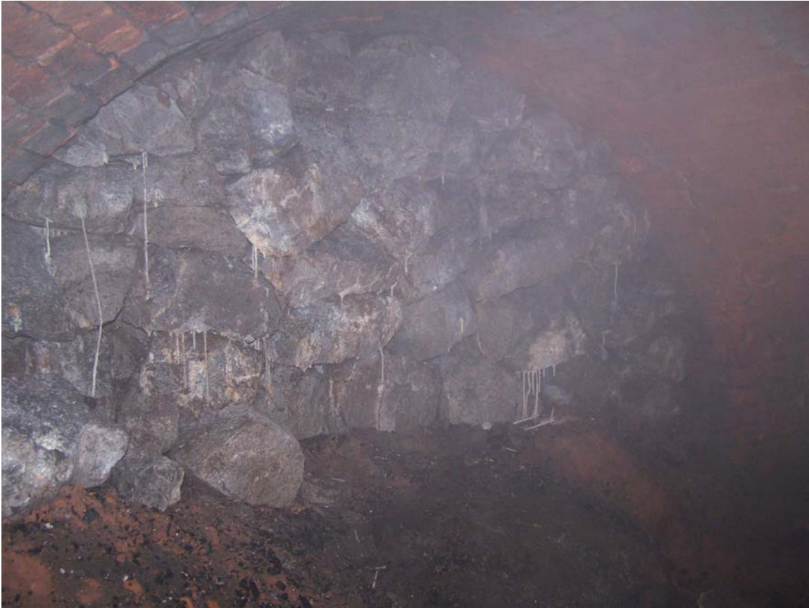
The stacked up stone closing off the shaft picture from the arched gangway. The canal entrance to this shaft is shown as the bricked up entrance earlier.
