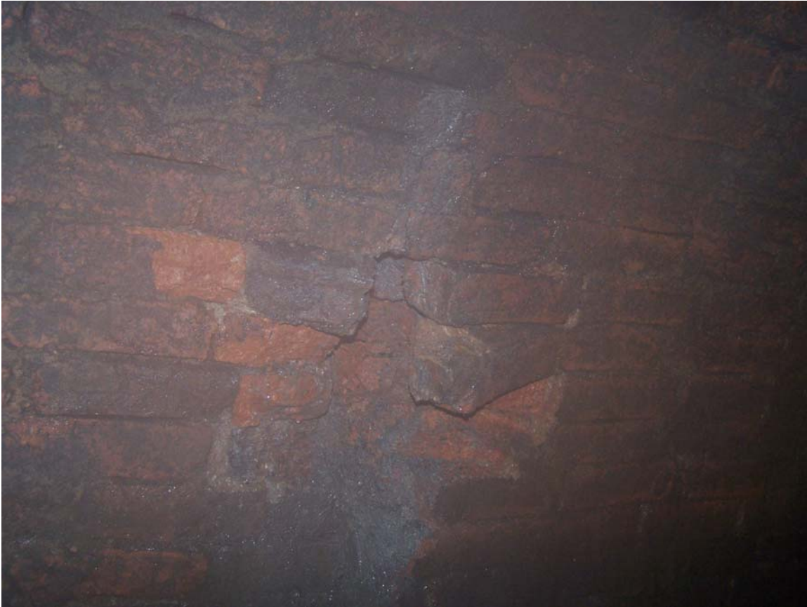
Damaged South wall just after Robin Witter's bulge.
