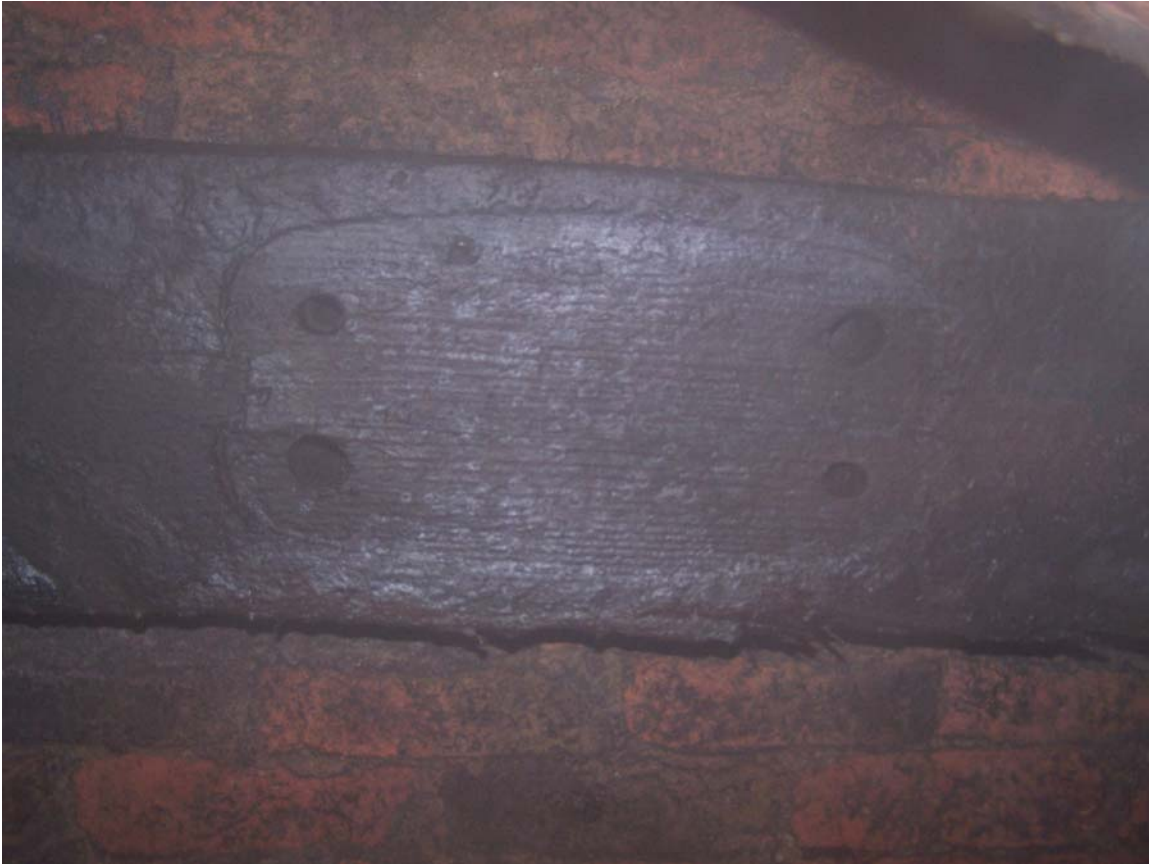
The roof shoring has these marks suggesting that the timbers came from a railway line.
