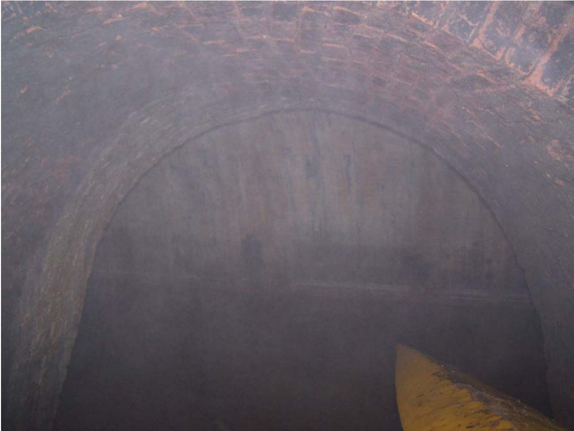
Looking out of the Arched Gangway to the Wide Hole. My canoe has been pulled up onto the wharf.
