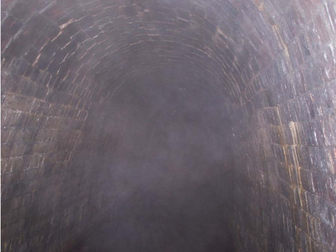
View from inside the adit towards the tunnel.
