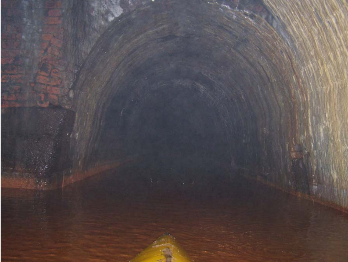
Looking back towards the Western Portal. Notice the small square hole on the North wall (right side of picture) about 2 feet above water level.
