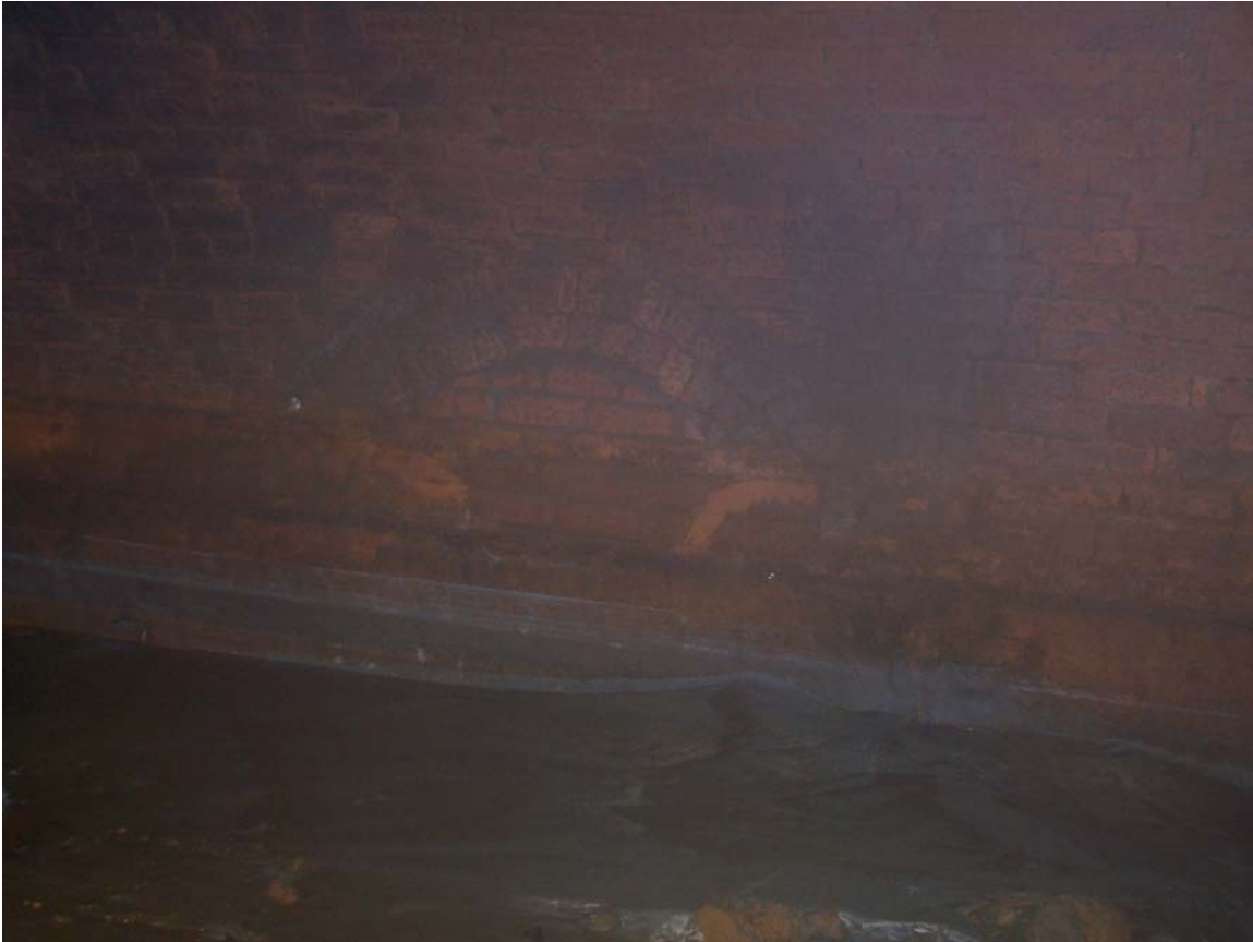
This bricked up arch is in the North wall just to the West of the Carr Pit exit and is labelled 'M' on the accompanying diagram.
