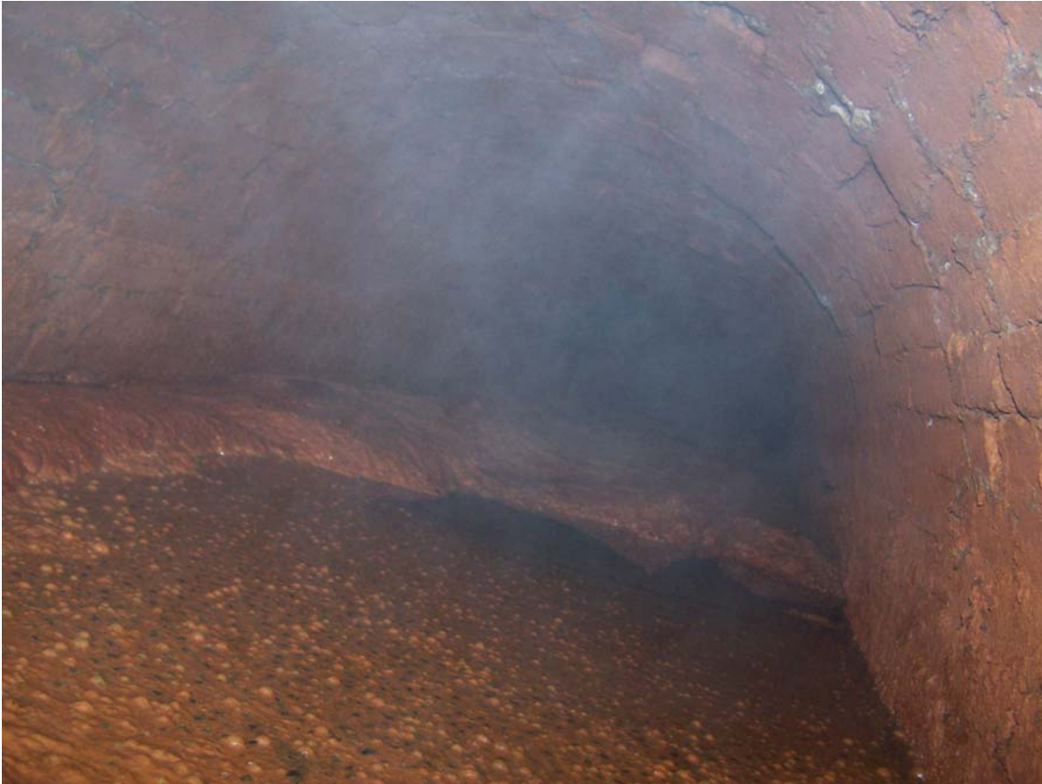
Looking South along the Carr Pit heading in the direction of point 'R'.
