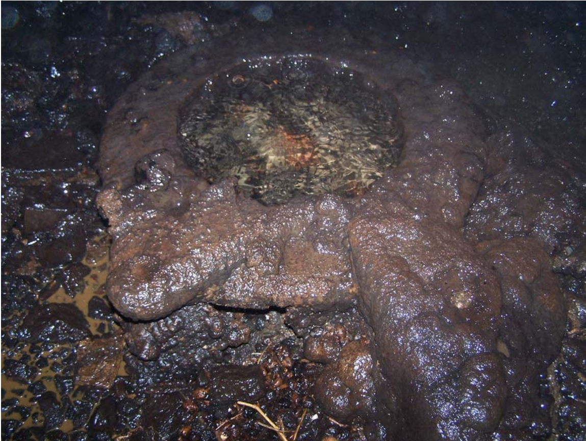
This flange plate is fixed to the floor of the blast receiver shaft. Labelled 'J' in the diagram.
