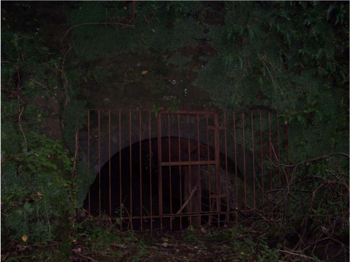
Closer view of Eastern Portal.
