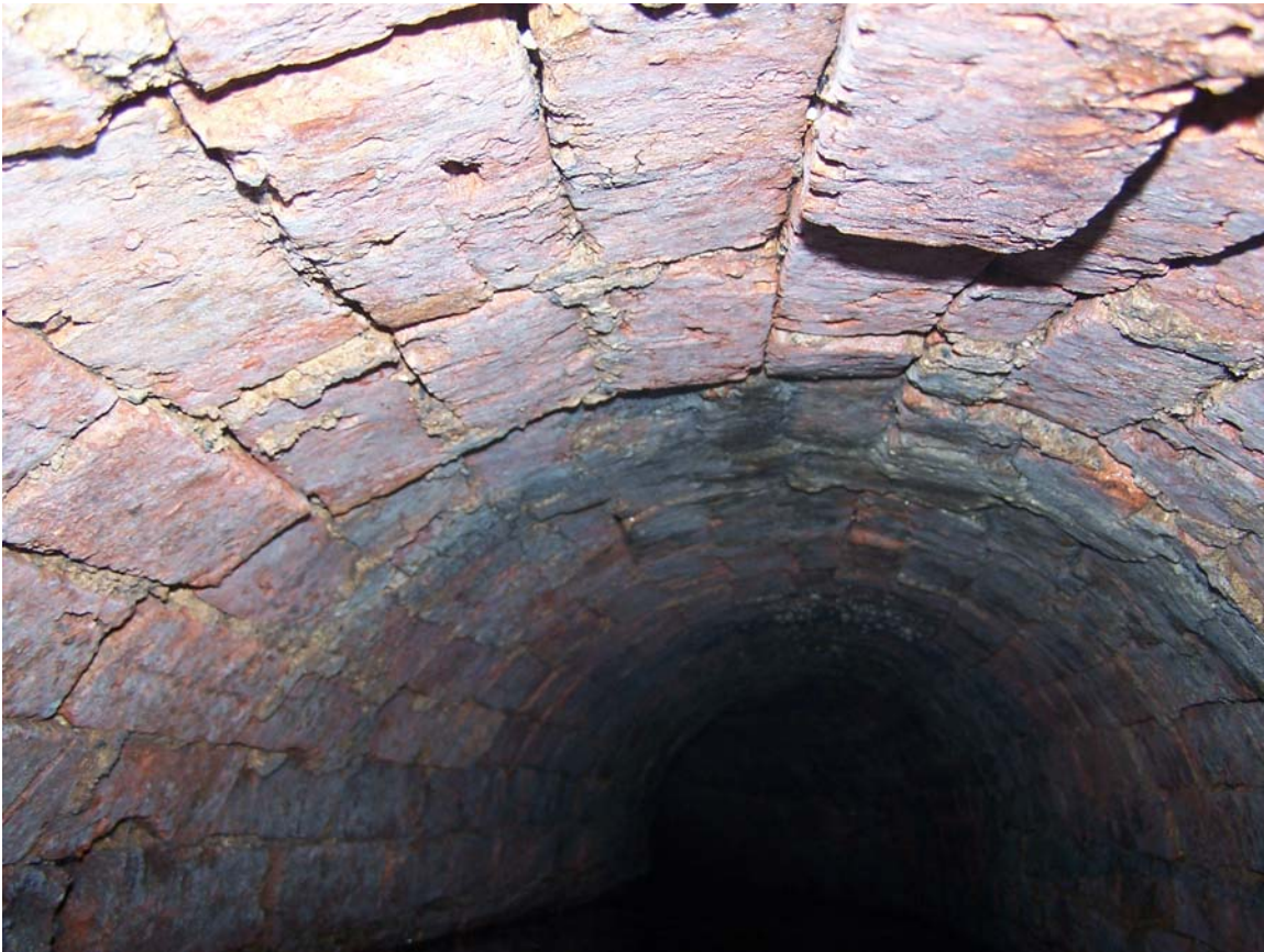
Inside the blast receiver tunnel. Photographed from point 'G'.
