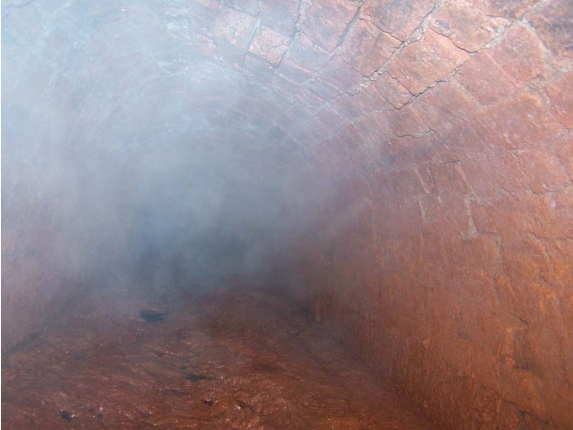
More Carr Pit Scum. This time photographed from the Wide Hole where the Car Pit heading enters at point 'L'.
