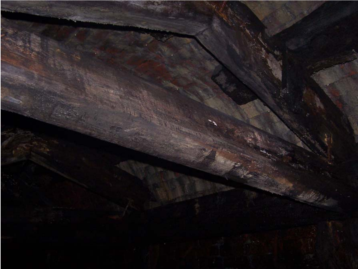
Shoring of the roof which might have allowed a narrowboat to pass.
