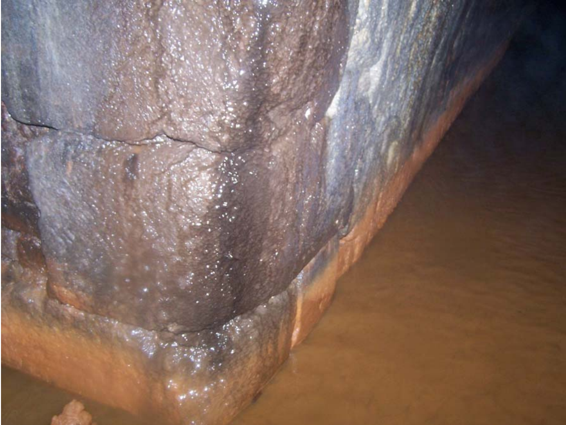
Close up of the masonry bumpers on the corner of the tunnel entering the wharf. Labelled point 'J' on the "Shaft under Blast Receiver" diagram.
