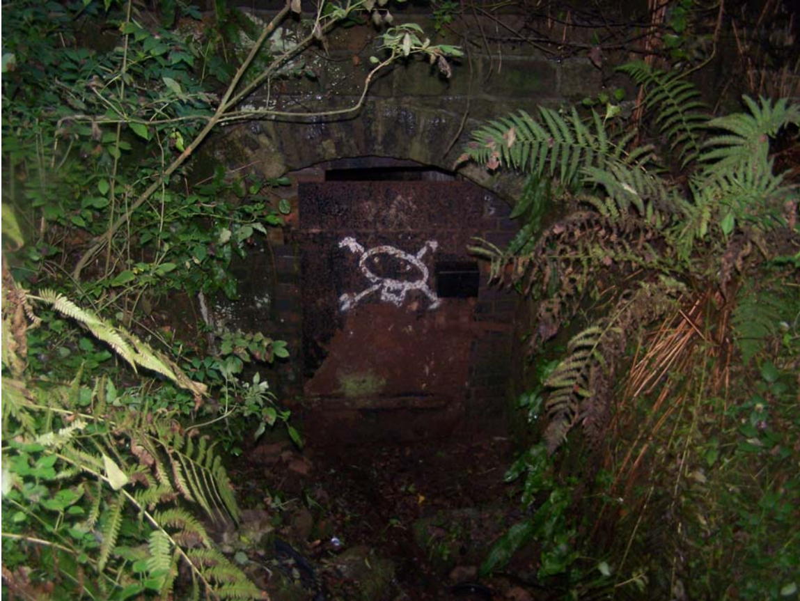
The entrance to Butterley Reservoir Adit next to Butterley Reservoir. This has a good quality lock.
