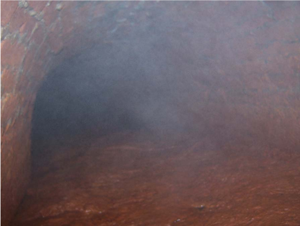
The Carr Pit heading looking towards point 'S', viewed from point 'Q'.
