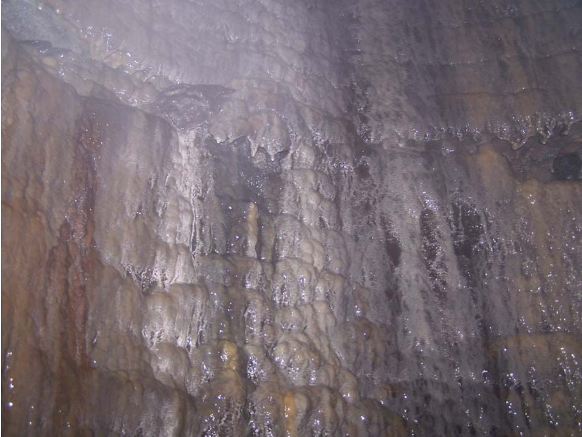
Flowstone on the wall of the loading shaft which is between 6' and 6' 6" not 7' wide.
