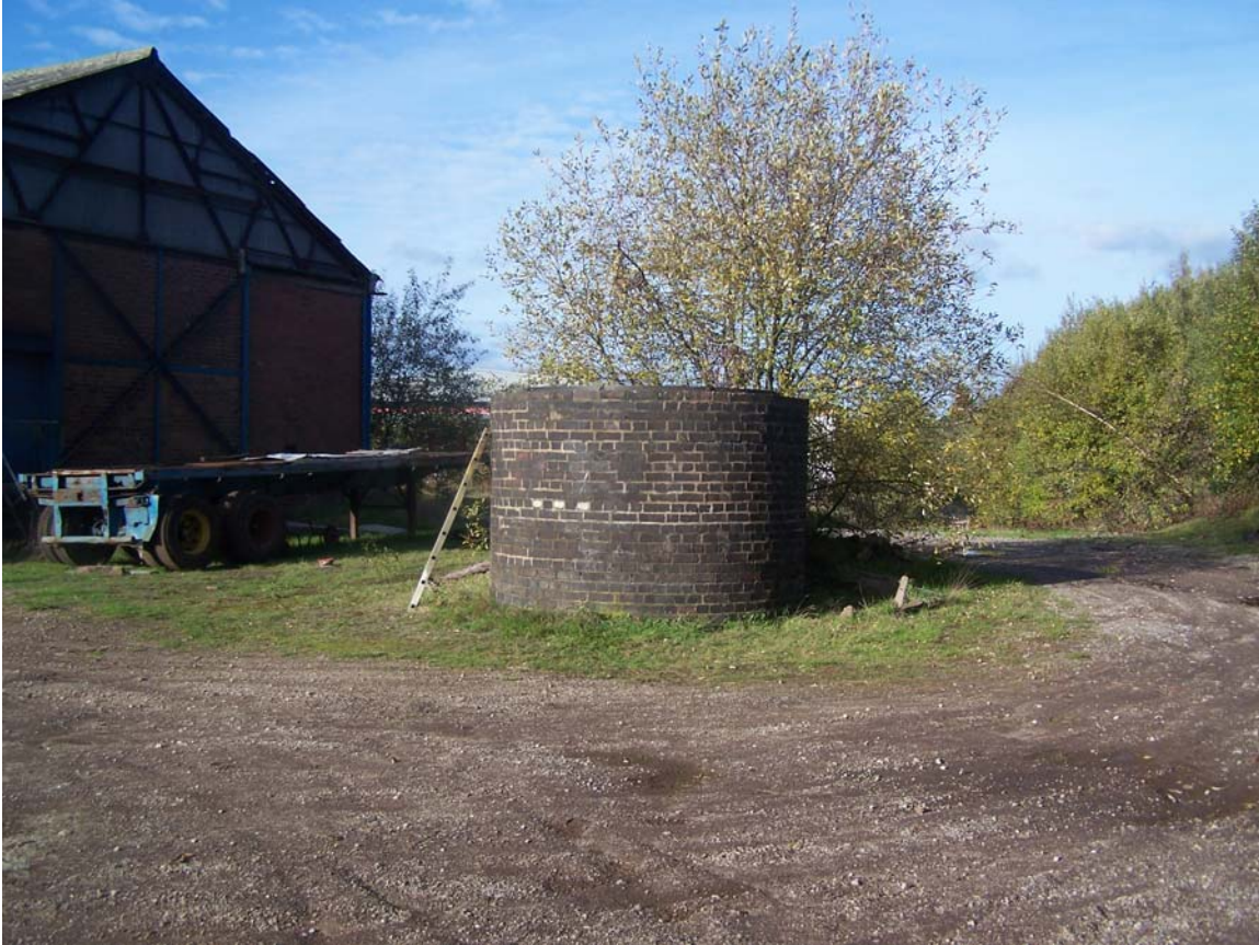
Shaft One at the surface has an iron grill across the top to prevent access. Someone has left a convenient ladder for photographers.
