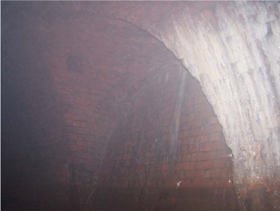
The bricked up entrance next to the main wharf. Labelled as point 'E' on the preceding drawing. The drawing also has a detail of this entrance.
