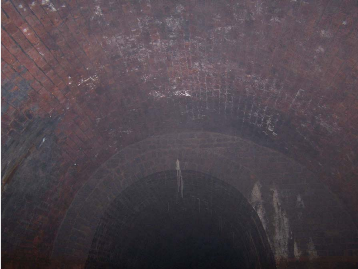
The brickwork put in when the Wide Hole was shortened.
