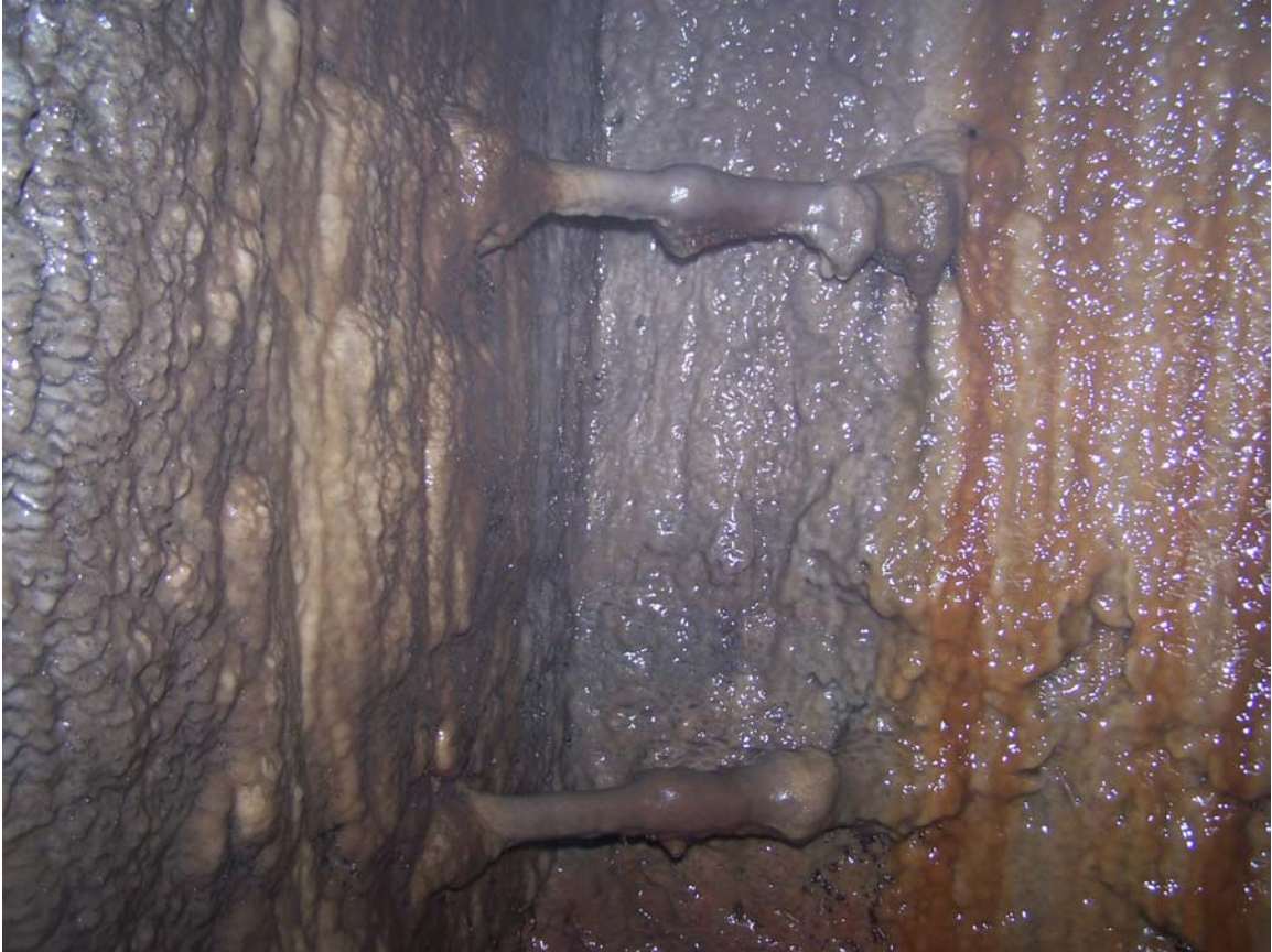
The Steps at point 'C'.
