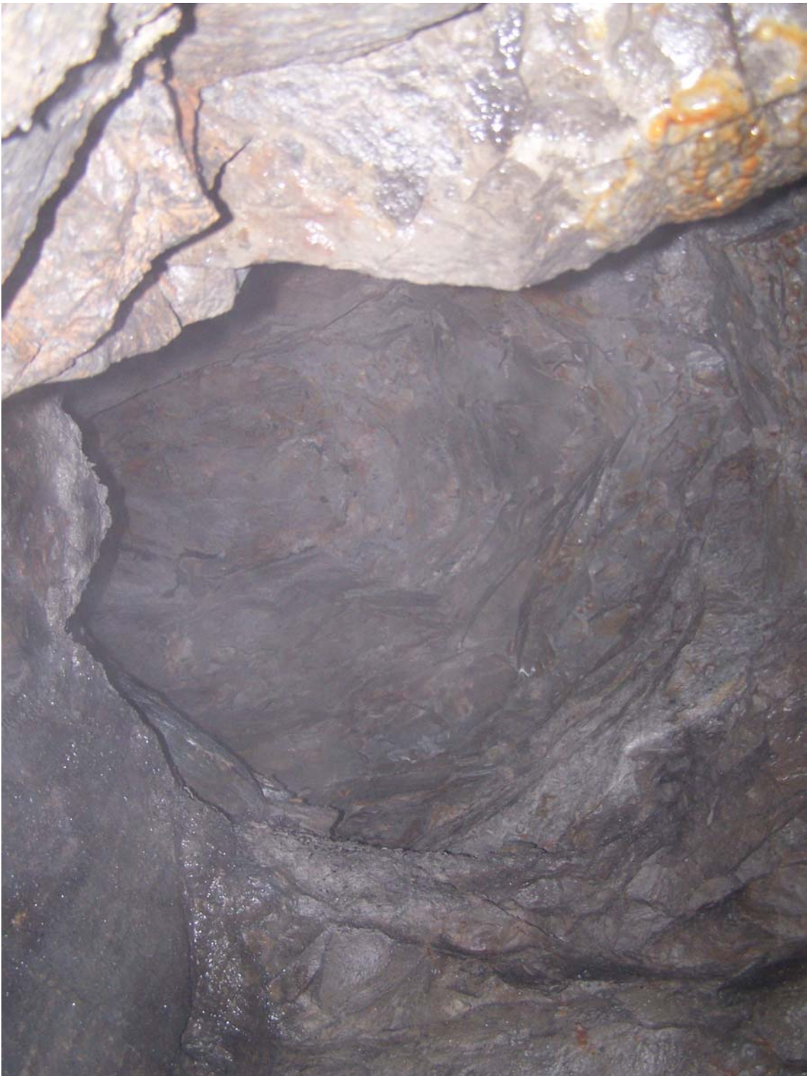
Looking up the old heading 'O'. This is not a horizontal view it is a view up the beginnings of a vertical shaft entirely in virgin rock, the siltstone earlier mentioned. About 20 feet of this shaft is visible from the base.
