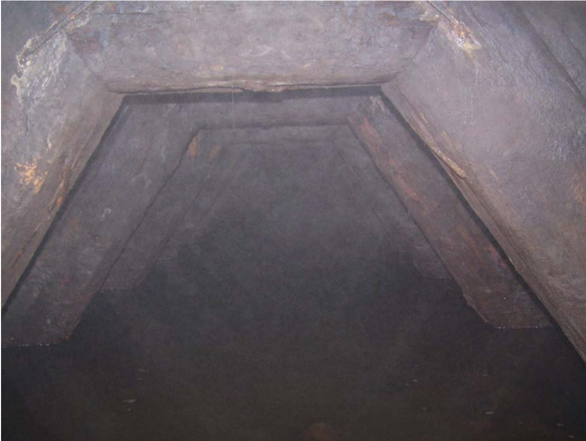
This is the style of shoring just before the collapse.
