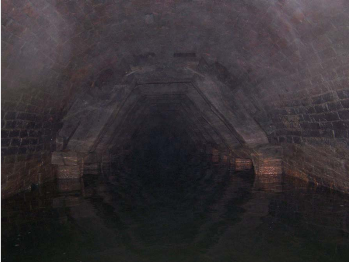
Third set of shoring starts at about chain 6.
