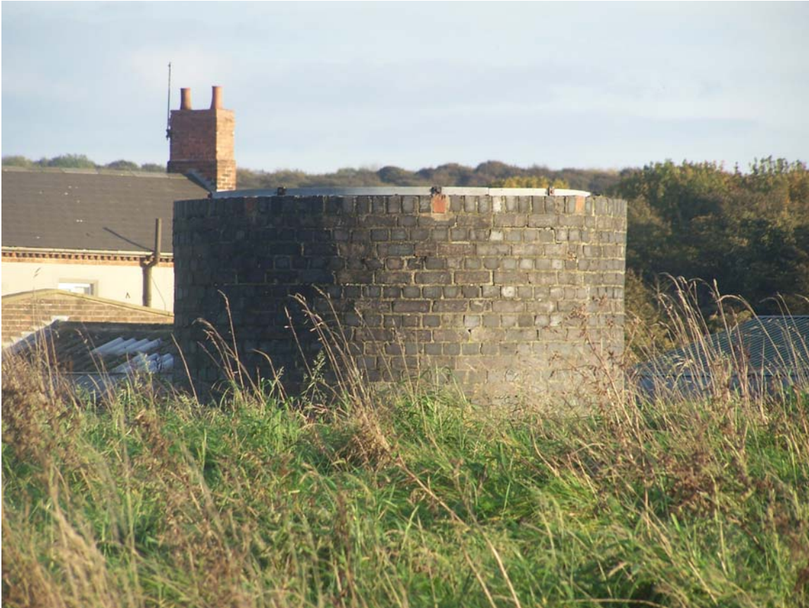
Shaft Four at the surface on the other side of the Coach Road. 53 degrees 3.487' N, 1 degree 22.917' W.
