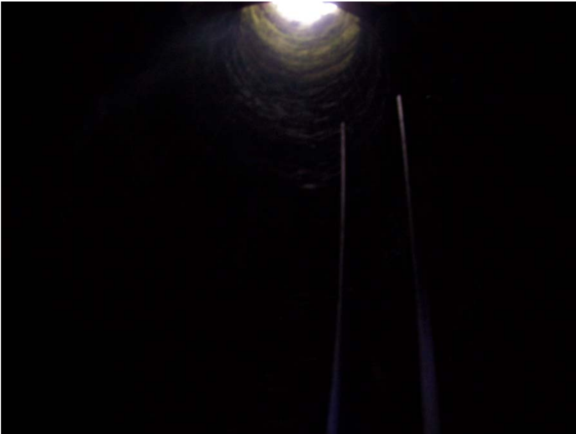
Daylight can be seen up the airshaft.
