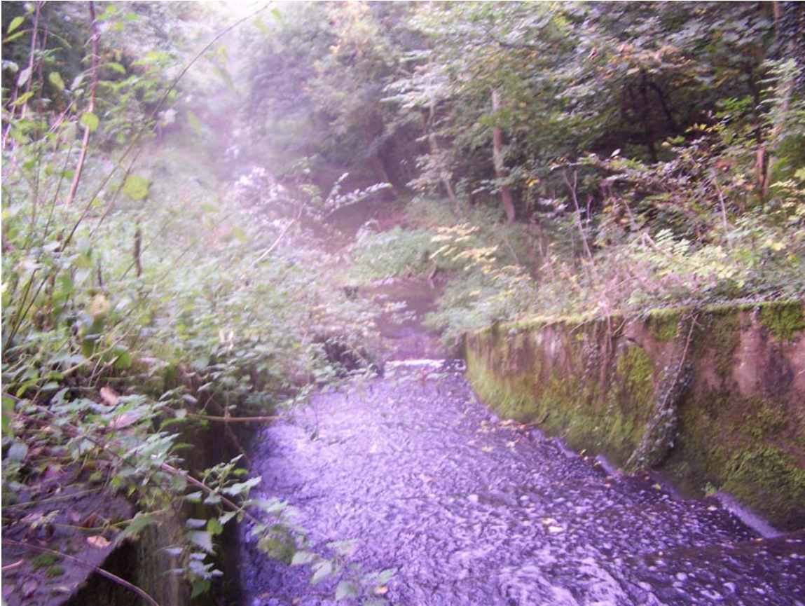
Water flowing down the spillway to the right (North) of the tunnel portal when facing the portal.
