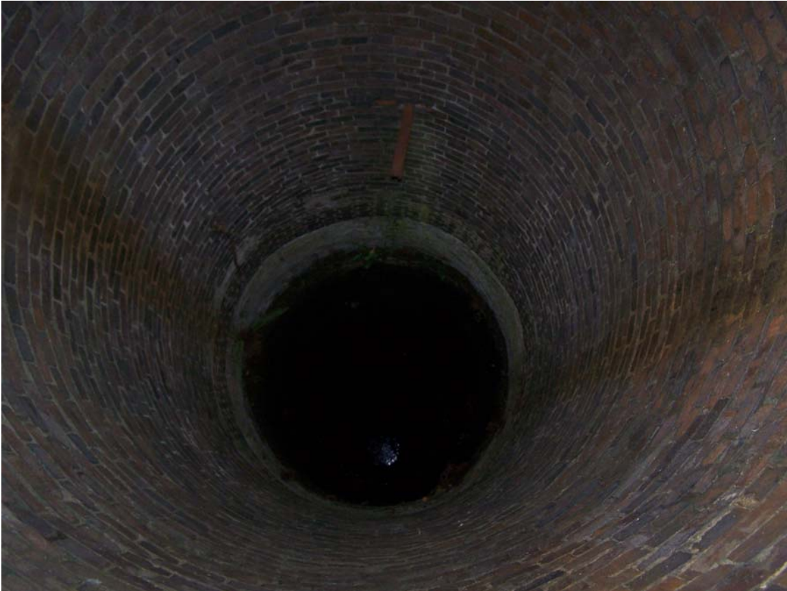
Looking down Shaft Two. Water is visible at the bottom.
