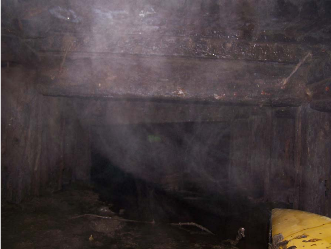
Looking backwards after passing the first shoring at Chain 3, the Eastern Portal can be seen. There is not yet enough water to float the canoe.
