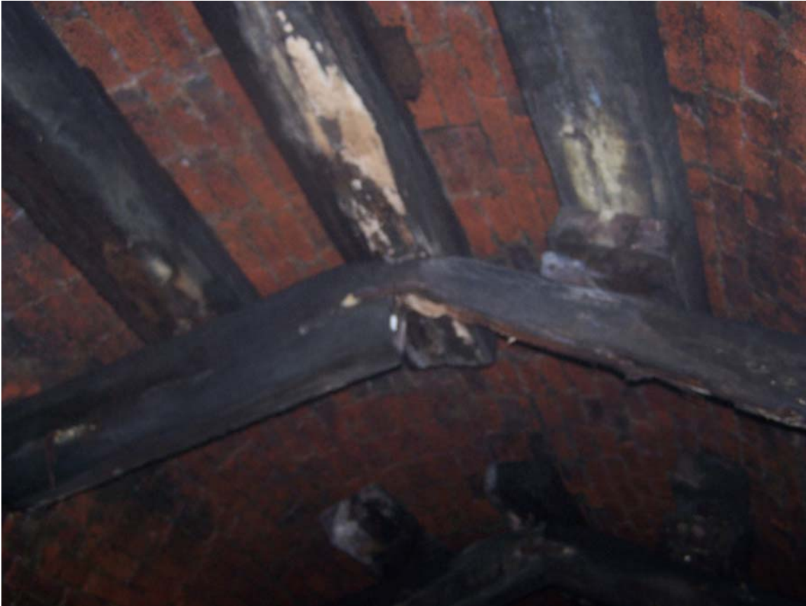
Close up of shoring showing slight damage to one beam.
