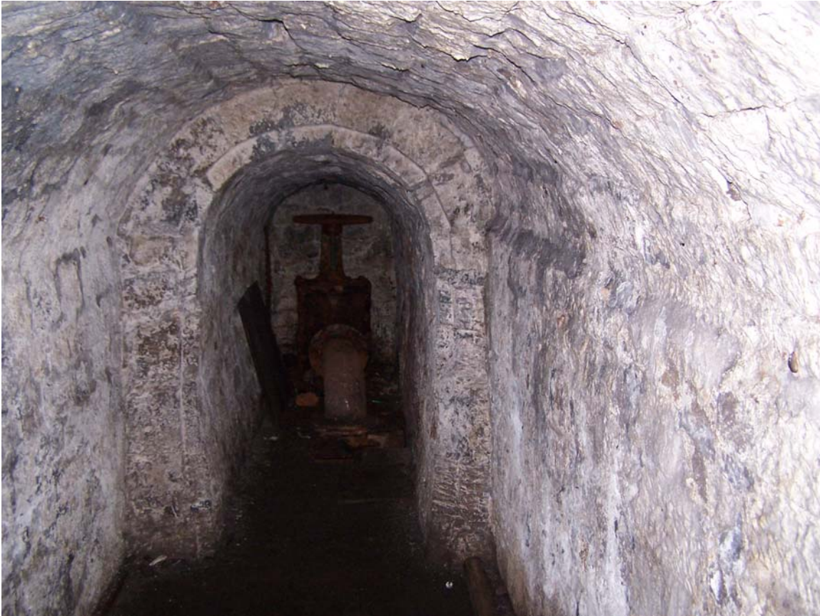
Photograph of Butterley Reservoir Adit Valve taken over the top of the locked door.
