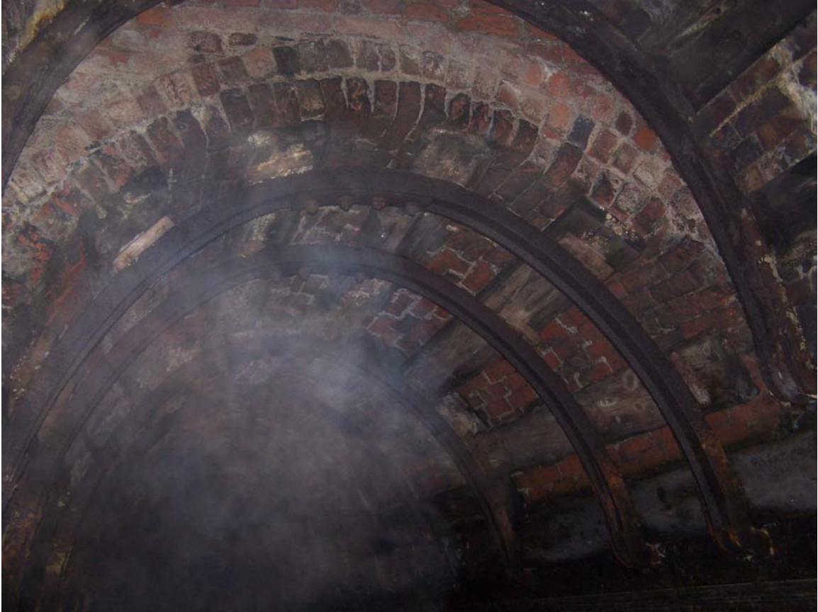
Bolts at the top of each iron arch.
