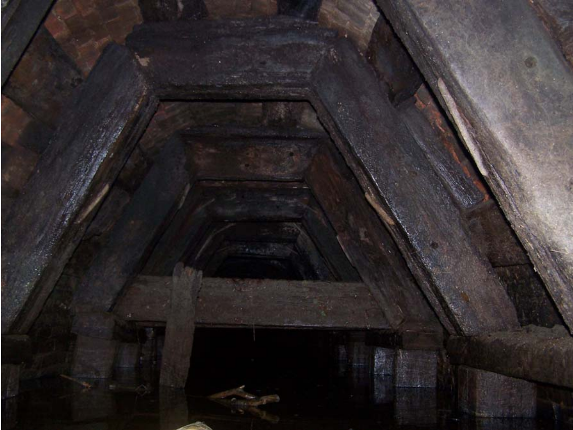
Second set of shoring in reasonable condition just before Chain 5.
