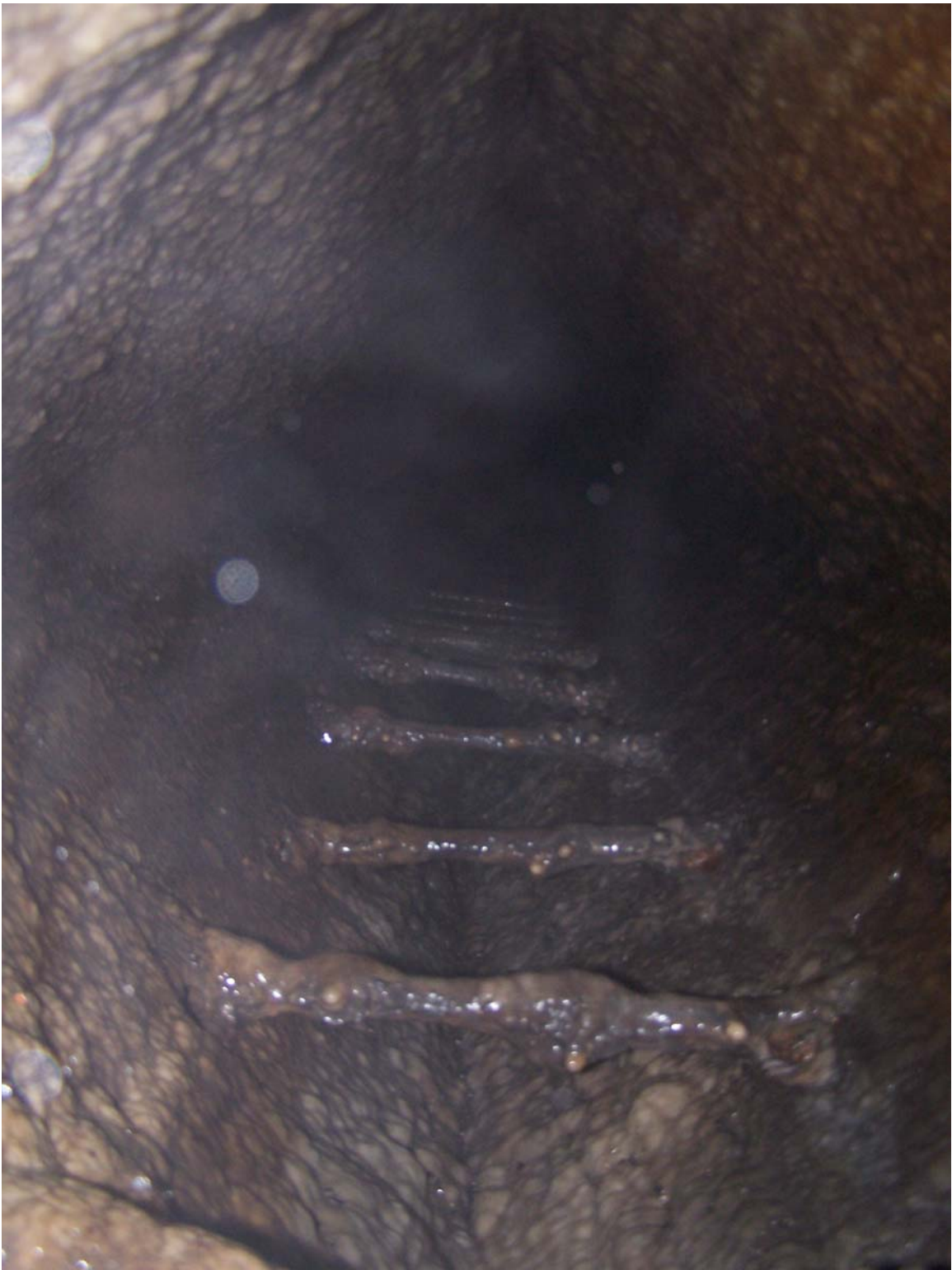
The ladder leading upwards from point 'C'. The 1915 Wide Hole drawing shows that this ladder leads to the base of the most westerly loading shaft. There are twelve steps 14 inches apart.
